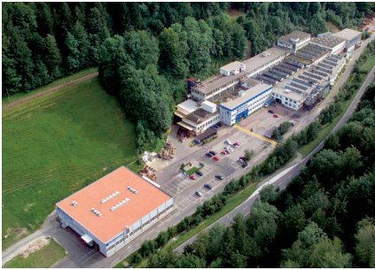
Wolfensberger's headquarters. In Bauma near Zurich, Switzerland, since 1924.
